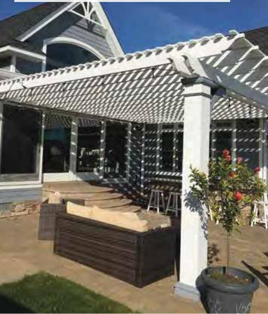
16x14 Structural Fiberglass Pergola, 10" square posts 9 ft tall, 2x8 rafters 16" on center
